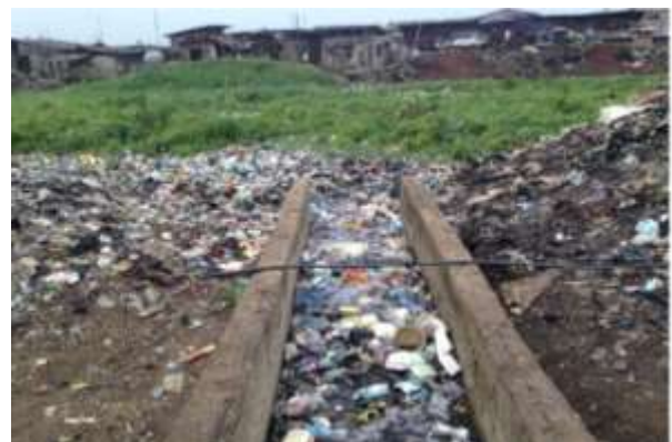
Plate 6. Municipal solid waste blocked a point of discharge into canal at Badia, Ajeromi-Ifelodun Local Government Area, Lagos State, Nigeria (Source: Authors' Field Survey, 2014).
